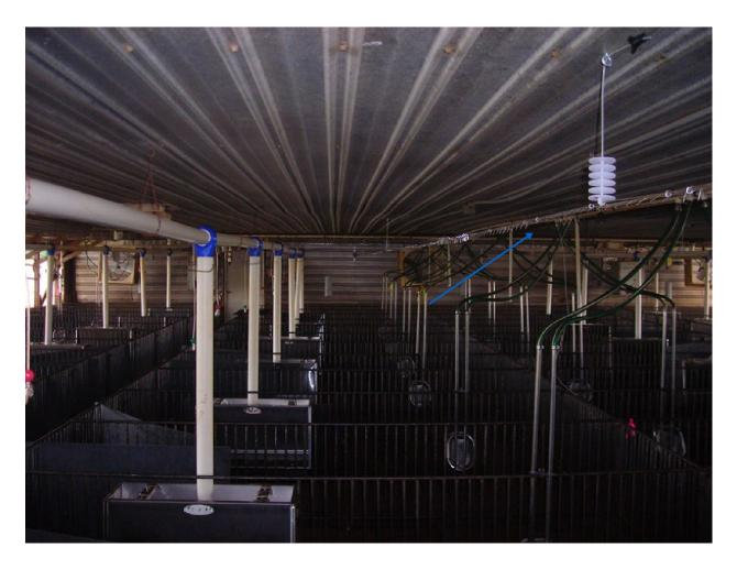
Our patented stainless steel corona points are attached to a stainless steel cable, which is stretched across the length of the production room. The corona line is connected to the lift system cabling via specially designed ceiling insulators spaced regularly along the length of the corona line. When the lift system winch spools cable, the ceiling insulators are pulled through the lift system cable support eyelets which, in turn, lift the corona line closer to the ground plane.
