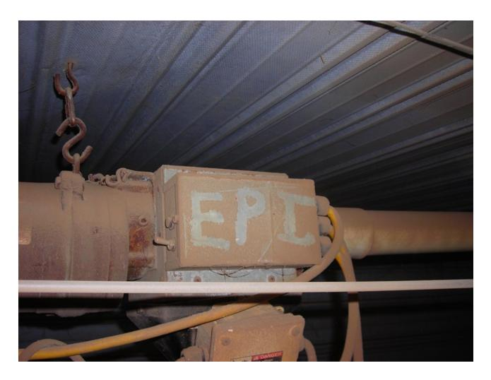
Another photo in the same room shows dust collecting on the feed motor. The EPI System requires a paradigm shift in thought about room cleanliness. **Dust collected on surfaces is much superior to dust suspended in the air.** Removing dust from the air enhances ventilation and reduces stress on the respiratory system, allowing pigs to grow faster. Again, this photo was taken after only two days of EPI System operation.
