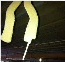
A thick dust layer can be collected, as shown in these photos taken inside this lowa wean-to-finish barn. **This 12 gauge wire has attracted a 1" diameter layer of dust.** When the animal production phase has been completed, wash and clean the room as normally done. When the EPI System is turned off, nearly all the components may be power washed.
