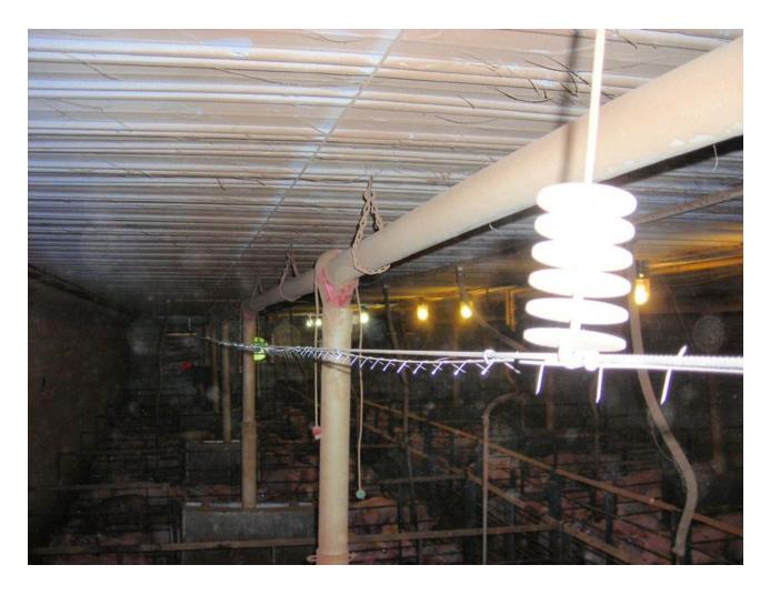
Polarized dust particles collect on the nearest grounded surfaces first, as shown on the ceiling and feed pipe. This EPI system had only been operating for two days in the swine nursery production room pictured. Collected dust is no longer available in the air to cause stress on the animals' respiratory systems. This allows the animals to grow faster. **EPI air is the best ventilation enhancement in decades.**
