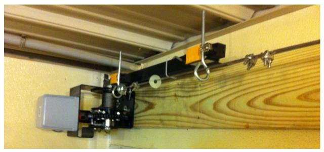
Stainless steel wire cabling is installed on the surface of a ground plane (usually the ceiling) and feeds to a central automated winch that lifts the corona line closer to the ground plane. This patented system maintains the ion flow of the EPI system to optimize the delivery of ions over time.
