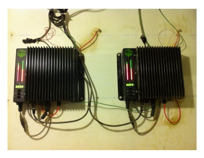
The power supply is mounted inside, or outside, the production room. Common 110-220 Volt, 50-60 Hz electric service is required. **The maximum wattage draw of one power supply is approximately 100 watts.** Specially designed red wire delivers the ions to the corona lines. Gray wires communicate with the automation switches and motor.
